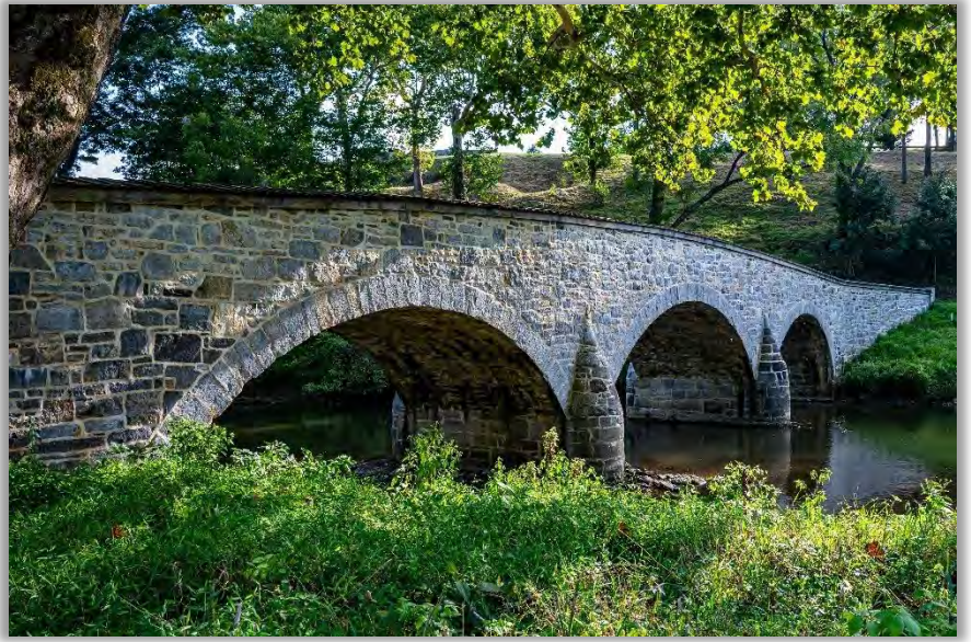
Historic Chapel in Elkton, MD & Burnside Bridge ALSS | 2048601944 & 2216449541
