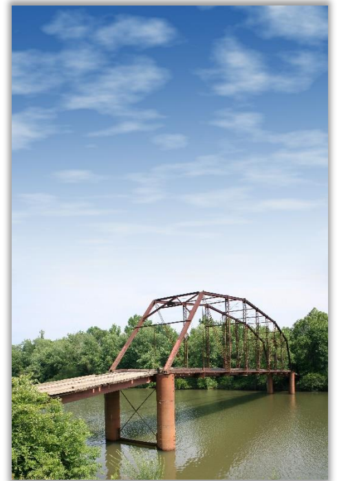
Little Rock Arkansas & Old Iron and Wooden Bridge in Arkansas SS | 1329642860 & ALIS | 609281
